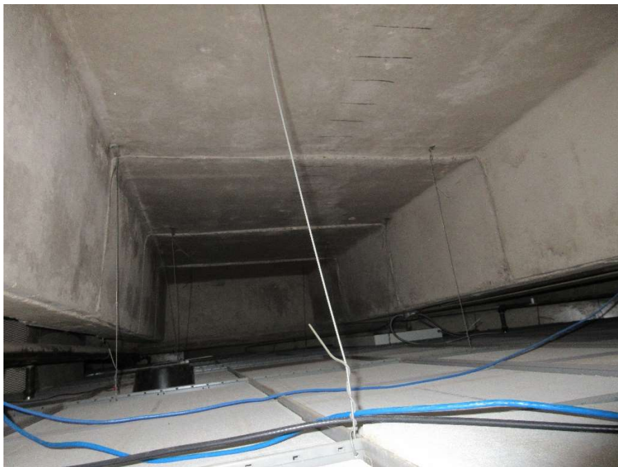
Photo 4 – Soffit of slab & joist floor system at Level 13
