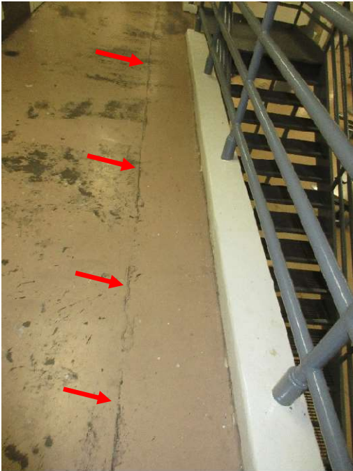
Photo 24 - Construction joint in slab top surface at Level 9
