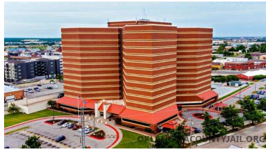
Figure 1 – Overall view of building (courtesy of OK County Jail)
