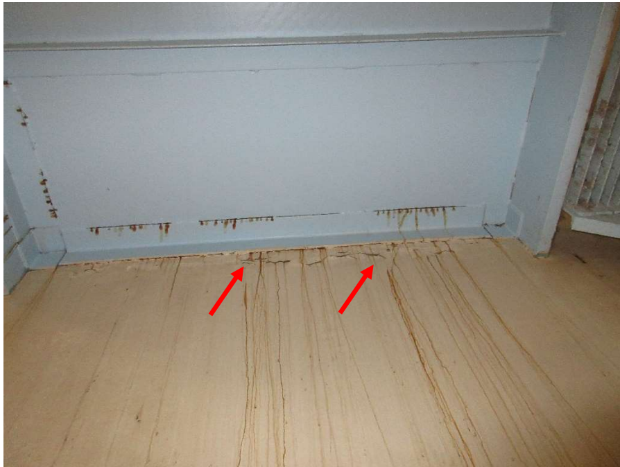
Photo 25 – Corrosion of edge framing at stair landing
