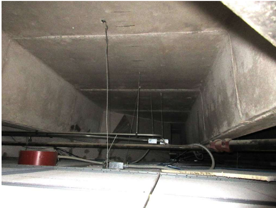
Photo 3 – Soffit of slab & joist floor system at Level 13
