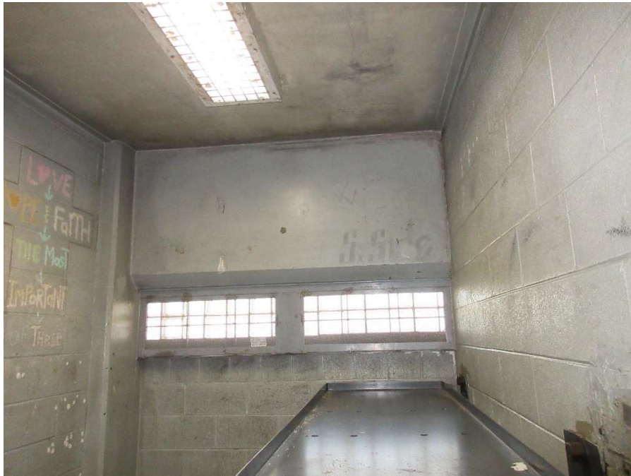
Photo 37 – General view of typical cell at Level 6
