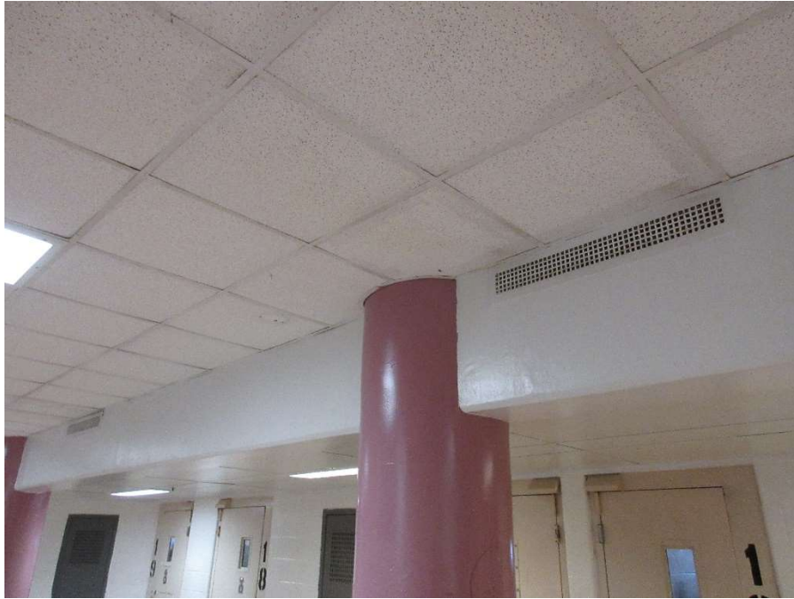
Photo 5 – View of large rectangular beams & round interior column at Level 13
