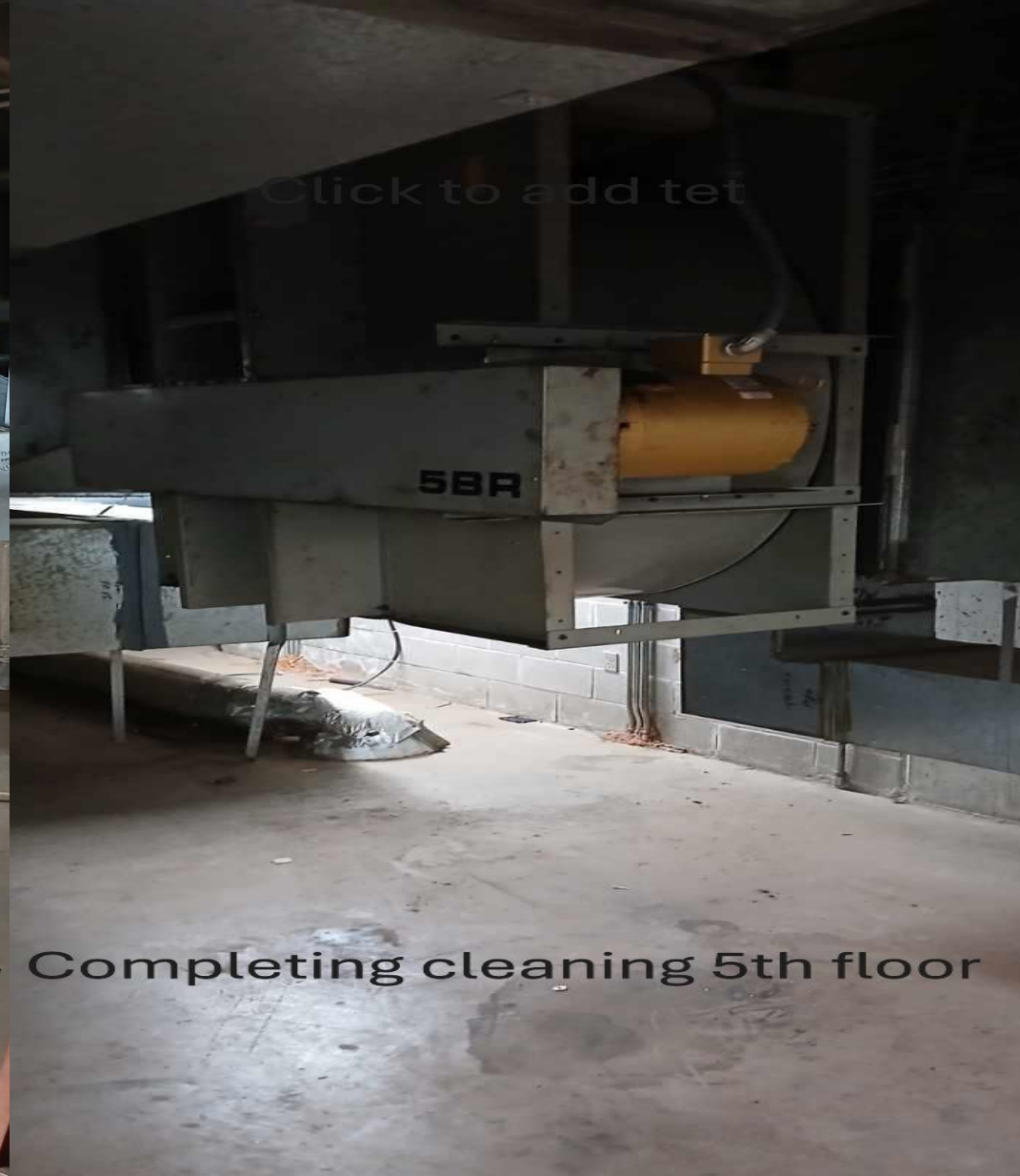
Cleaning 5th floor
