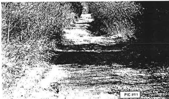
Narrow, one lane road; bar ditches silted full
