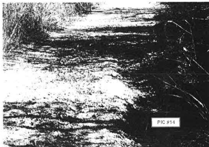
Deep rut eroded from storm water draining on road bed
