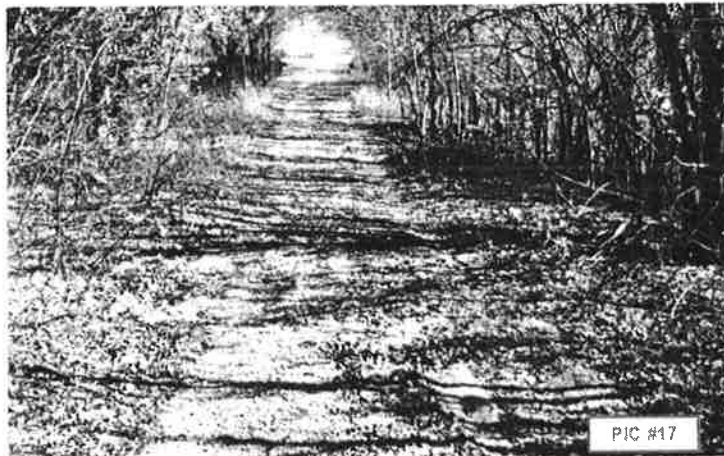
Example of silted bar ditches and lack of maintenance
