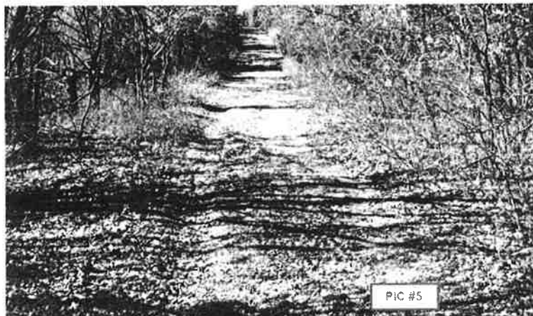
Bar ditches are silted full; storm water runs down road bed
